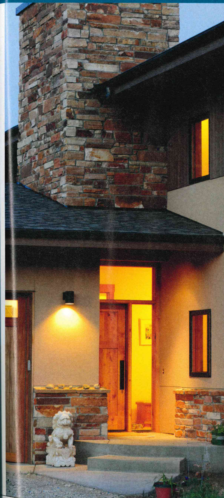
A faux-chimney can be used to house and camouflage an evaporative cooler as well as all mechanical room venting.
